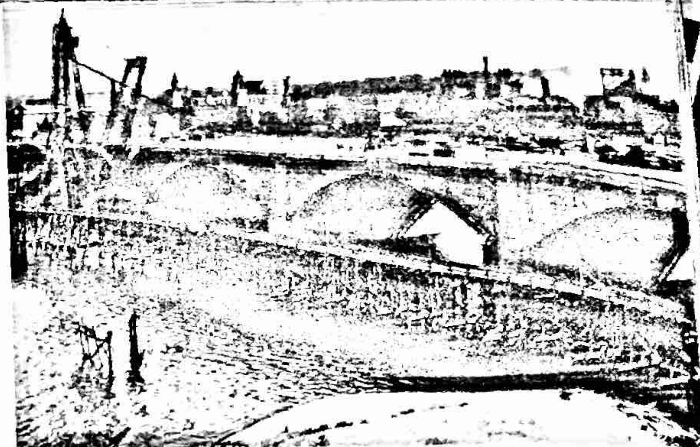
Bridge construction. Concrete hoisting tower (130 feet) shown. Concrete was transported from mixing plant on West Springfield side along a temporary wood trestle 70 feet upstream. Courtesy of the Lyman and Merrie Wood Museum of Springfield History.
