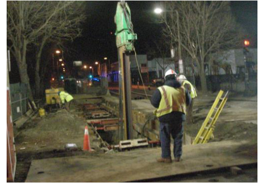
Crews drive piles as part of the Roxbury sewer separation effort.
