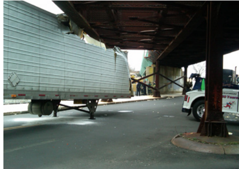
Wamsutta Bridge (before): The existing span arrangement and clearance over Acushnet Avenue had caused numerous accidents.
