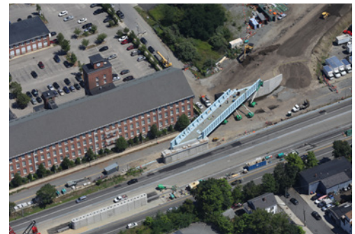
Wamsutta Bridge Precast Wingwall Erection (top) and Aerial View of Span 3 Erected (above)
