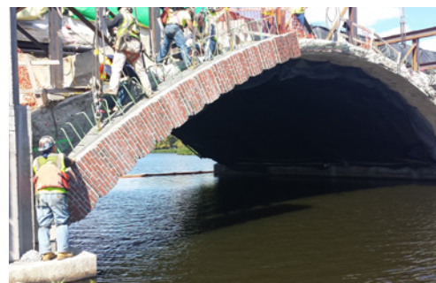
Construction of precast arch segment with brickwork
