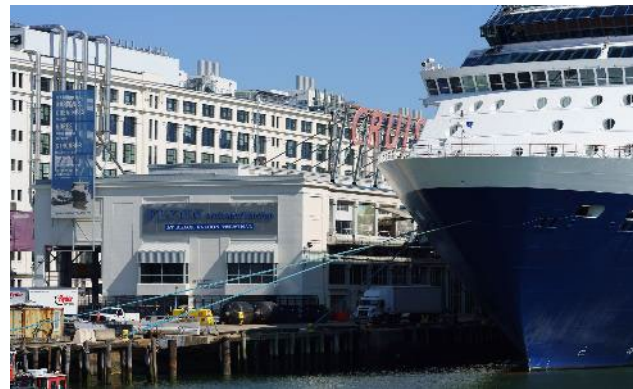
Cruise Terminal HVAC Upgrades (NZ) (on-going)
