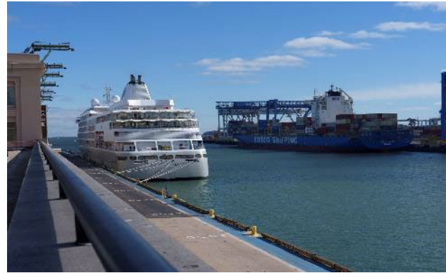
Cruiseport Pier Rehab (on-going)
