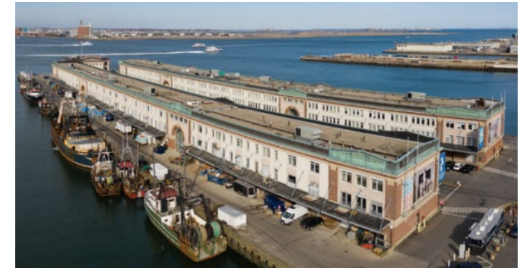
Fish Pier Roof (on-going)
