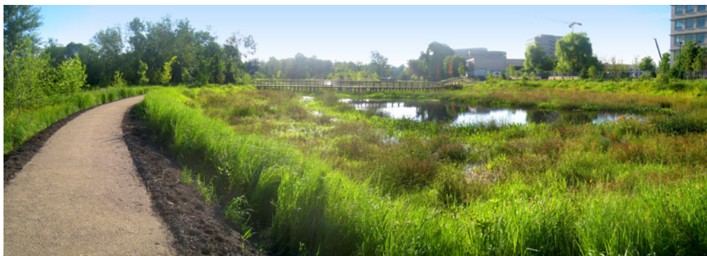
Stormwater from the CAM004 neighborhoods is conveyed to the Alewife Stormwater Wetland, where the water is stored and treated before it drains to the Little River on its way to the Alewife Brook.
