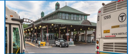
Bus Transfer Center
