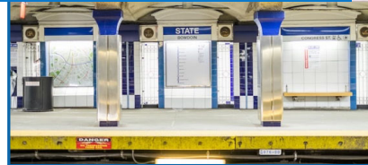
Underground Fixed Guideway Station
