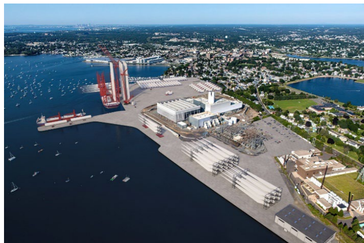
Figure 2.4-1 Salem Offshore Wind Terminal
