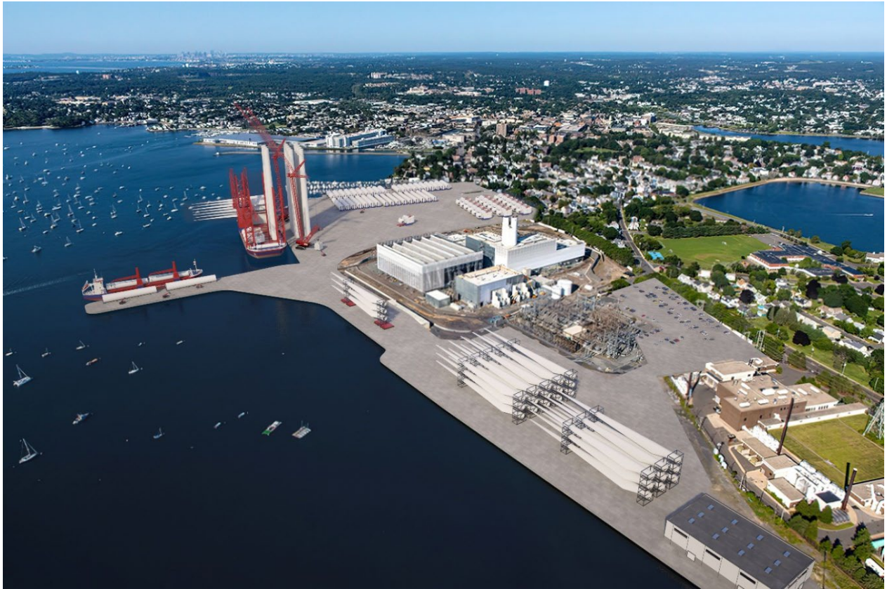
Figure 13.3-1 Salem Offshore Wind Terminal
