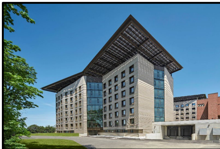
Massachusetts Veterans Home at Chelsea, rooftop solar array.
