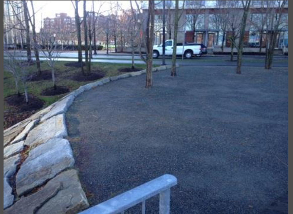
Use of pervious pavement to reduce impervious surfaces and promote infiltration.
