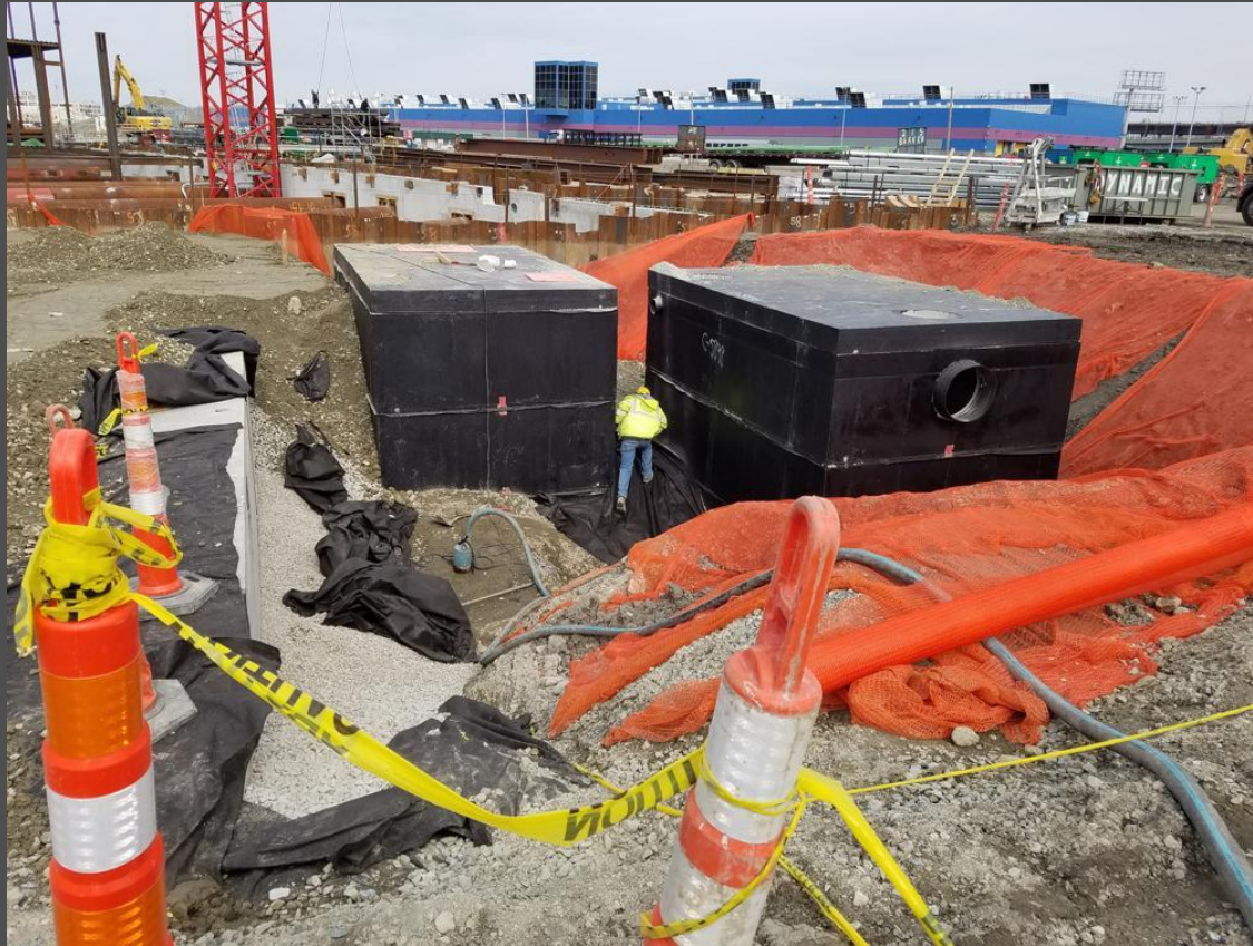
Cisterns for the collection of rainwater from roof runoff for irrigation.
