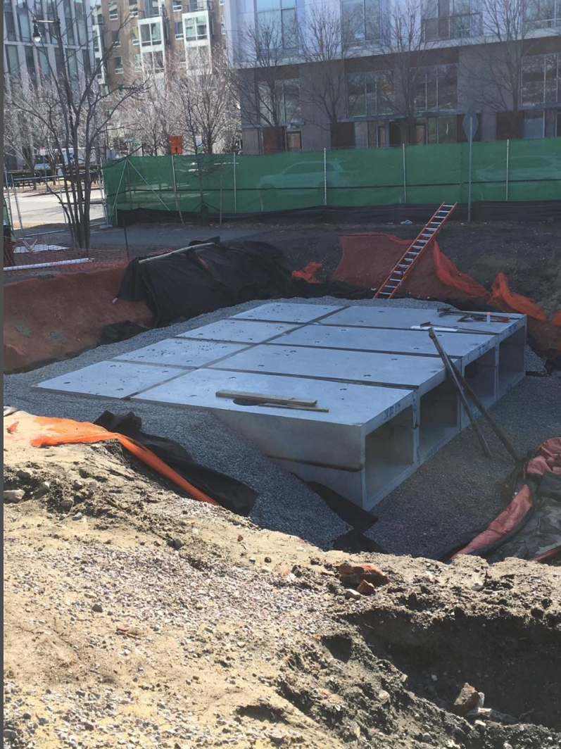
Installation of stormwater infiltration system within the open space network.
