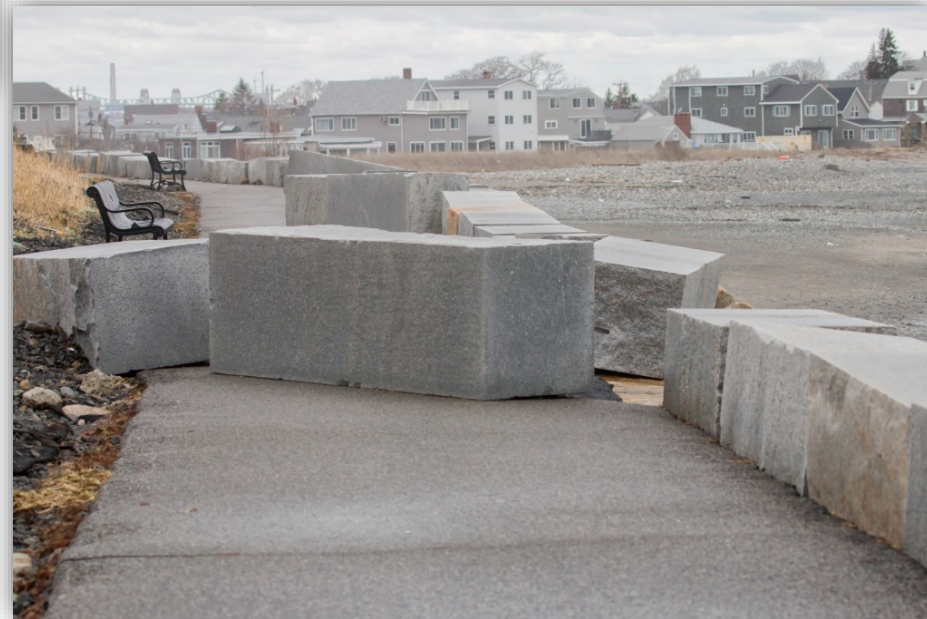
Fallen tree in front of historic pump station; granite blocks along public access were moved by waves
