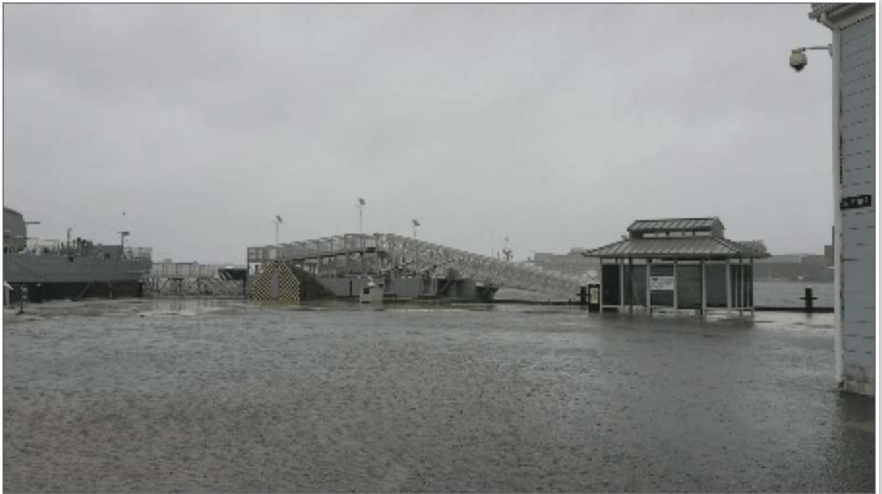
Pier One was flooded from overtopping of seawall
