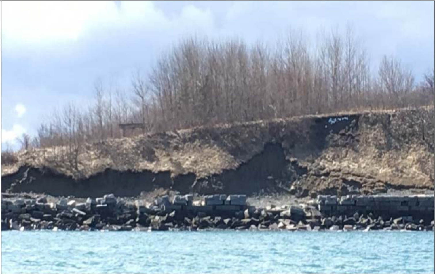
Looking southwest, showing continued damage to historic seawall and erosion of bluff that protects cemetery
