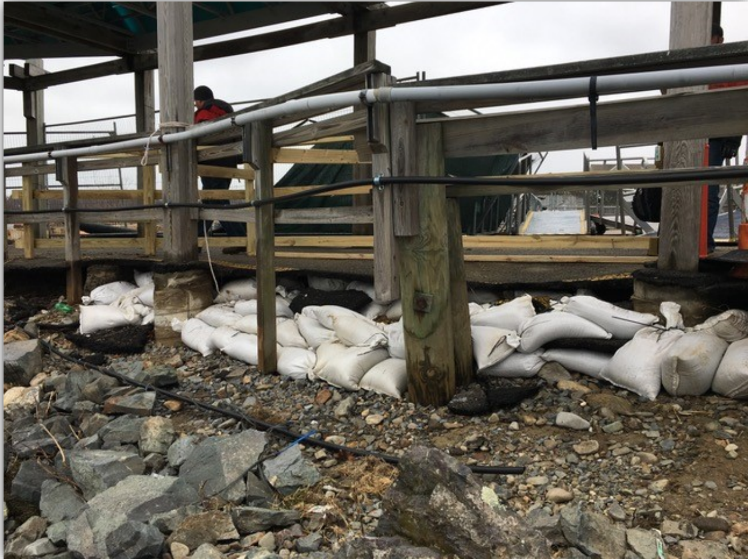
Undermined revetment and walkway
