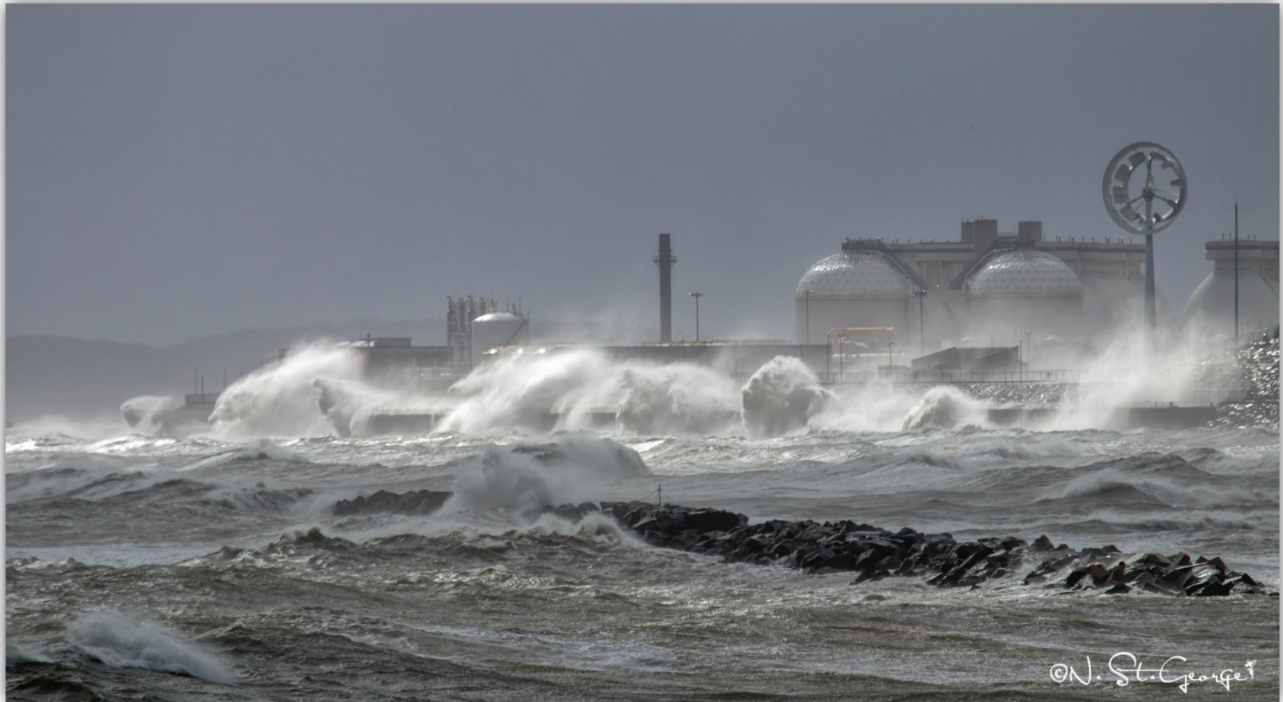
The seawall protects the island from storm surges
