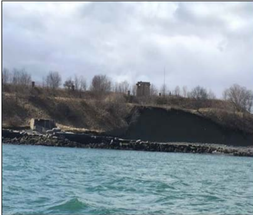
Looking south, showing continued damage to historic seawall and outer earthworks of Fort Warren
