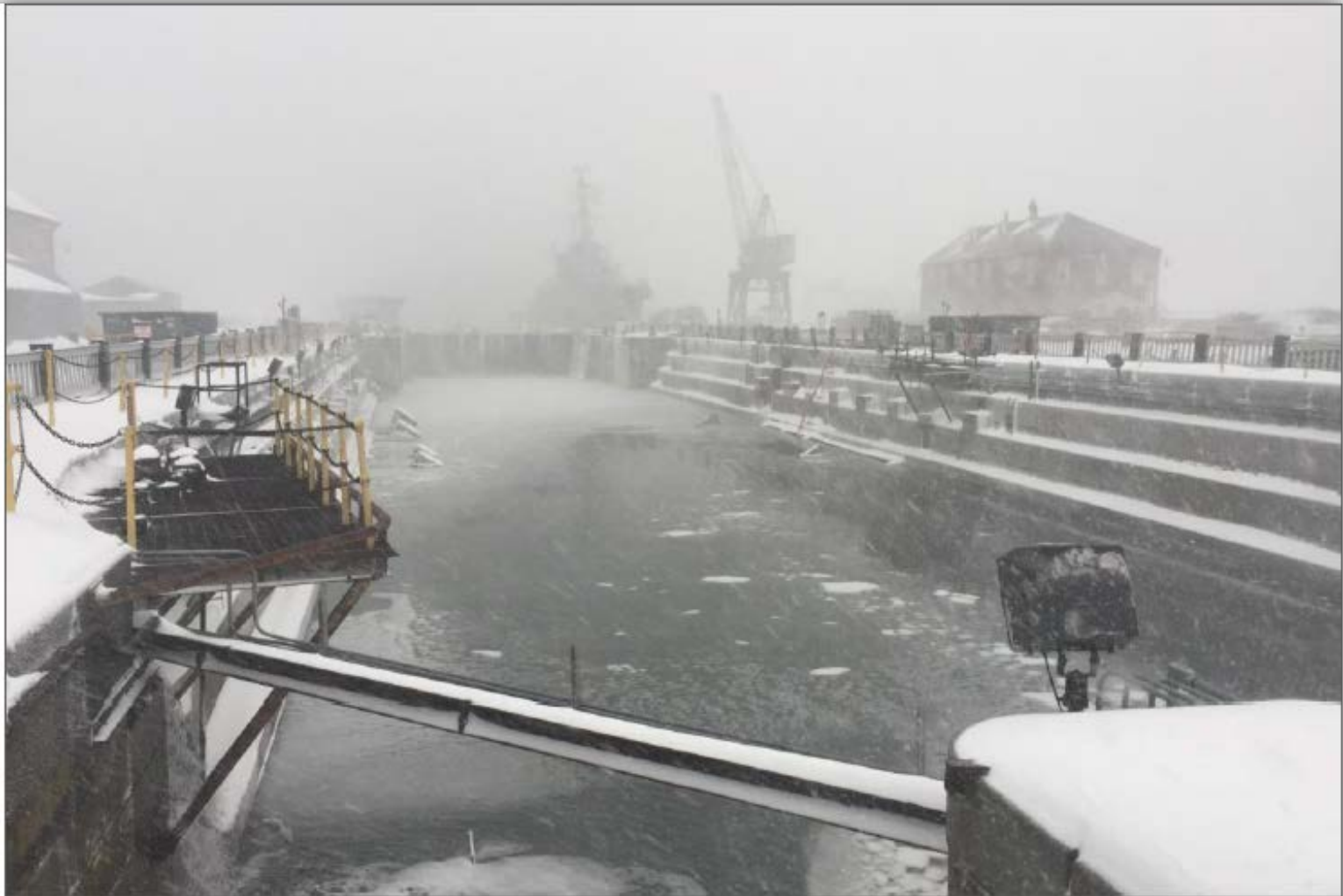
Dry Dock received 15 feet of water from overflow of caisson, overtopping and pump drains
