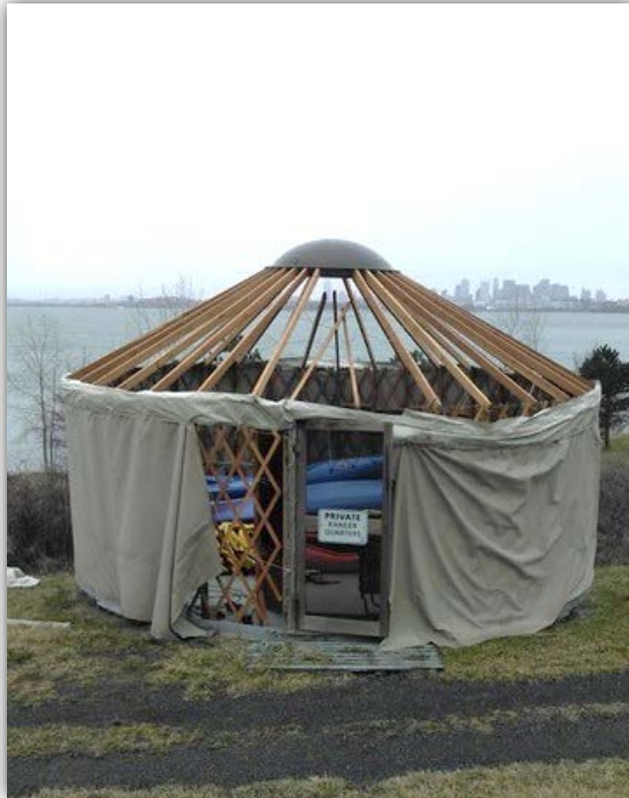
Damage to yurt
