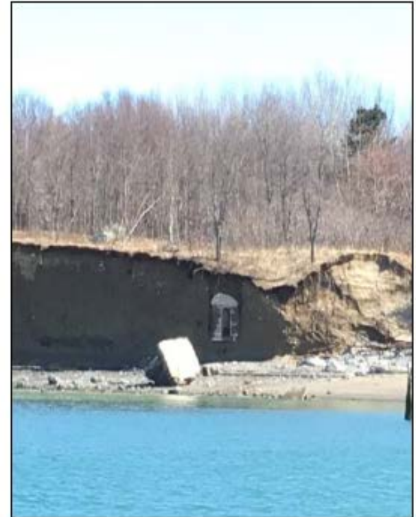
Looking east, showing perched doorway and tunnel entrance associated with Fort Standish coastal defense installation
