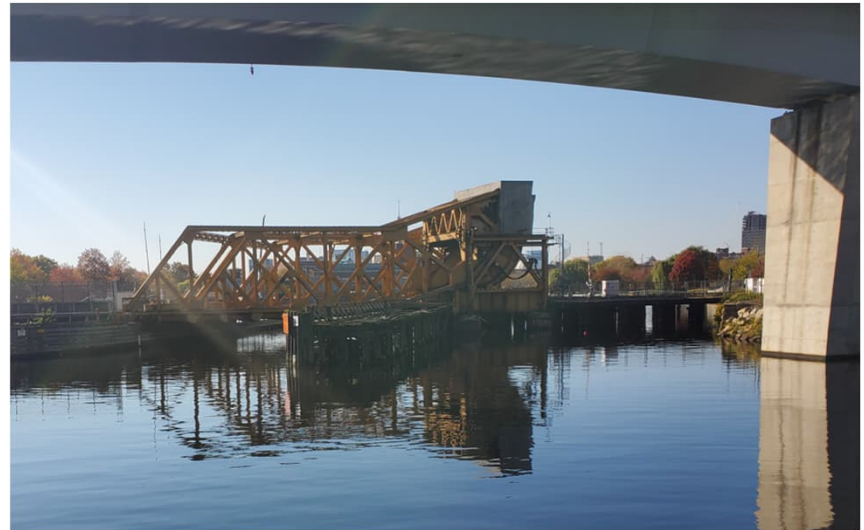
North Station Draw 1 Bridge Replacement
