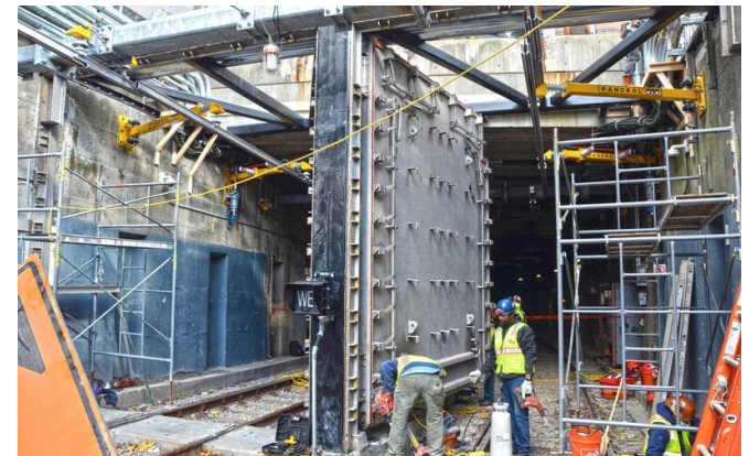
MBTA Fenway Portal Flood Protection
