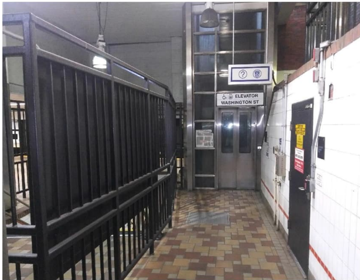
Downtown Crossing Station Accessibility Improvements
