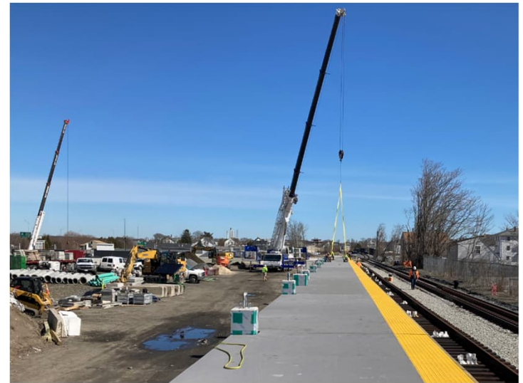
MBTA SCR Fall River Depot Construction
