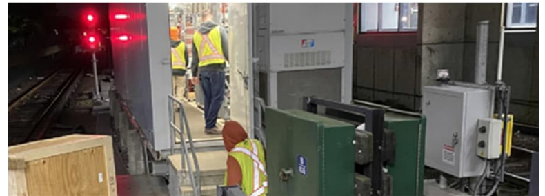
MBTA RLT Crew inspecting signal equipment
