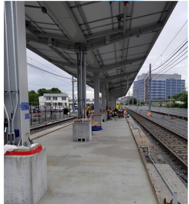
GLX Union Station construction
