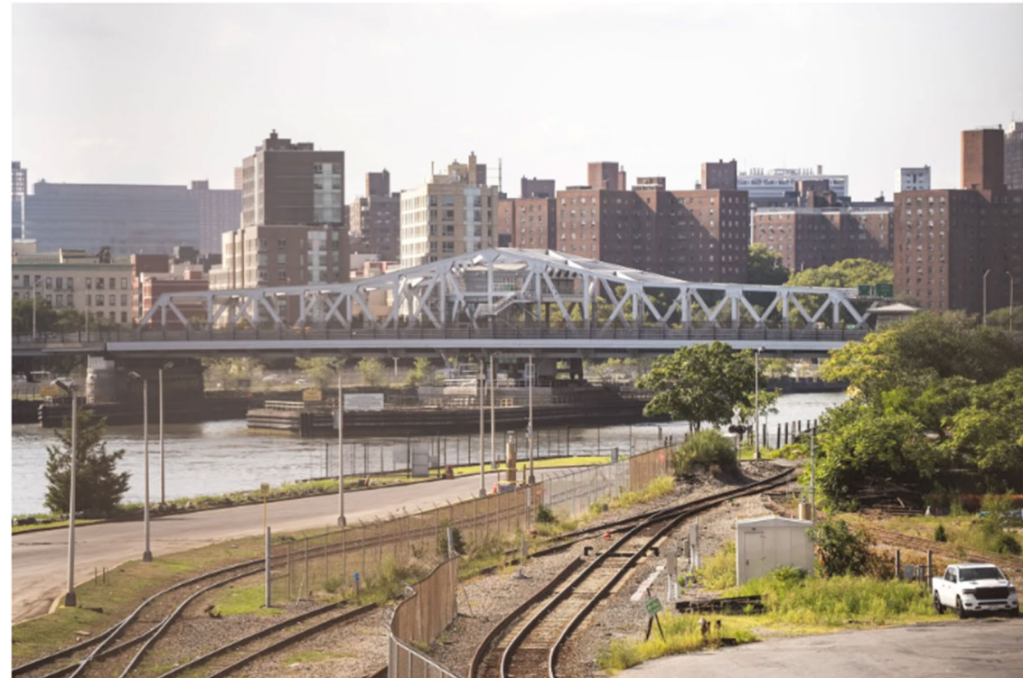
The Third Avenue Bridge, connecting Manhattan and the Bronx over the Harlem River. Earlier this summer, extreme heat caused a joint to expand and the bridge was stuck in its open position for hours. Graham Dickie/The New York Times
