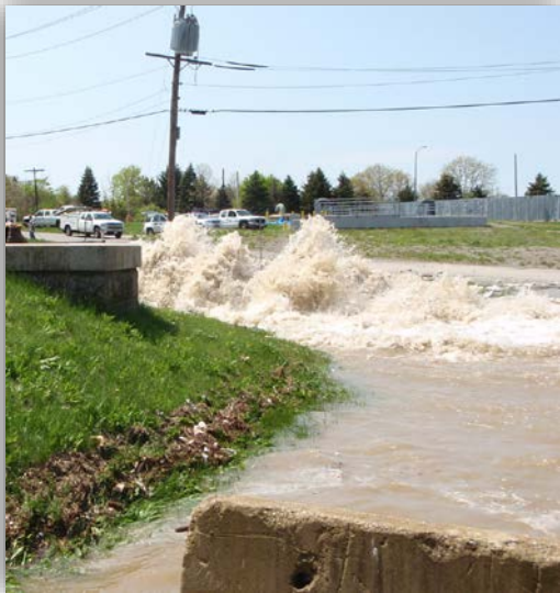
250 MGD flow at Shaft 5 break....
