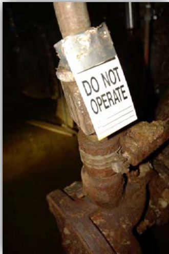
Shaft 8 PRV Chamber
