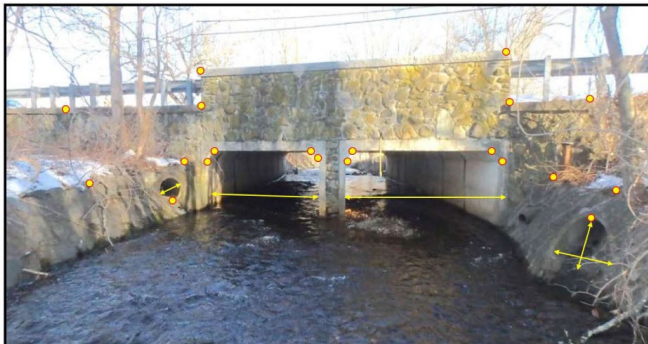
Figure 1.1.5-4 (a): Multi-Span Structure (Open Bottom) Survey Locations
