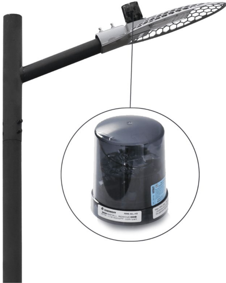
Example control node and receptacle
