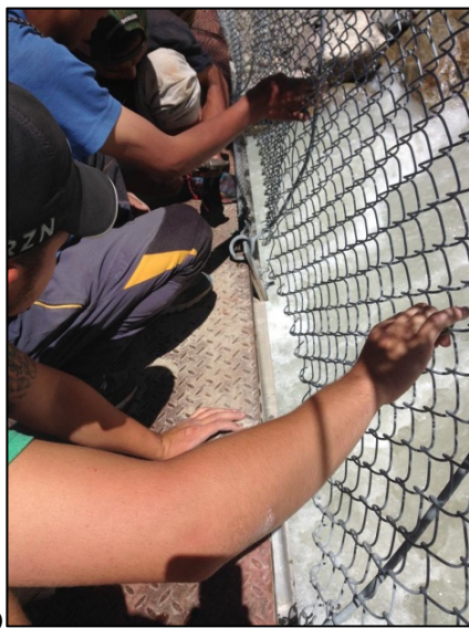
Figure 8 a) Threading the main cables through the hanger padeye loops at the deck b) Pulling the main cables through the hanger padeye loops.
