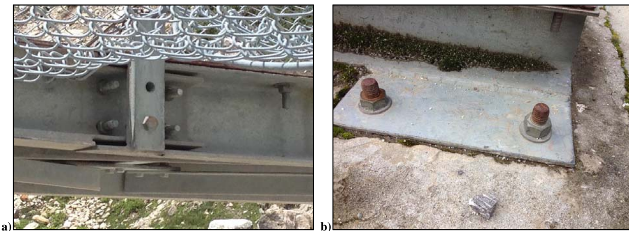
Figure 16 a) Detail of web connection of deck channels. b) Detail of anchor bolts at abutment.
