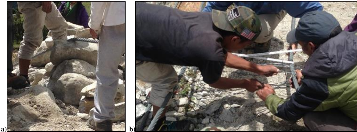
Figure 10 Secondary tensioning of cables. a) Using large stones to prop the cables. b) Securing pinched location with galvanized wire.
