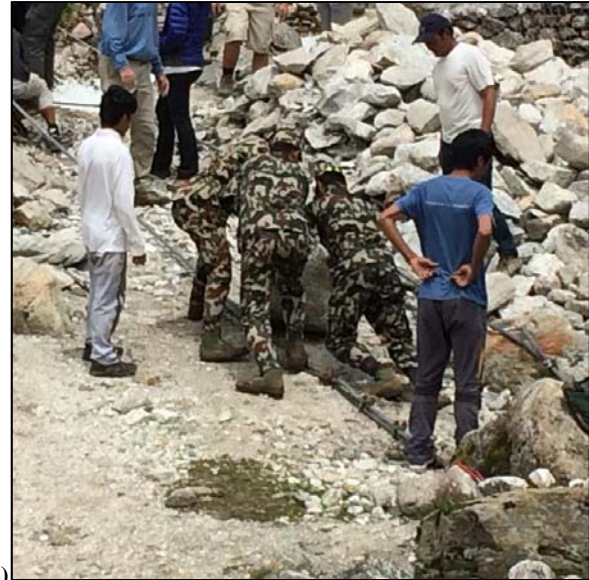
Figure 7 a) Clearing away the tower stones and releasing the main cables from the Yullajung anchorage b) Positioning large stones with the assistance of the Nepal Army.
