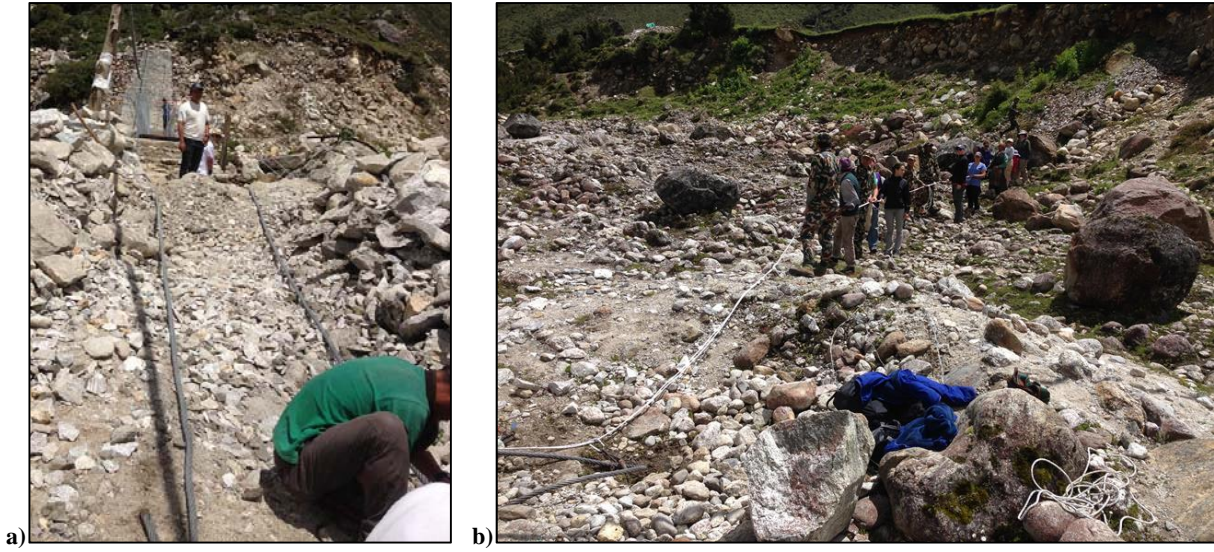
Figure 9 a) View of main cable alignment from Yullajung anchorage. b) Preparing to hand tighten a main cable.
