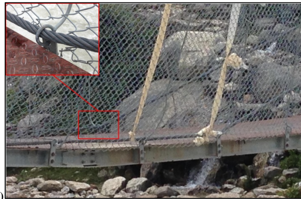
Figure 13 a) New signage near entrance to bridge. b) Detail of main cable at deck level. Note the threading of the main cables through the padeye loops of the hanger rods.
