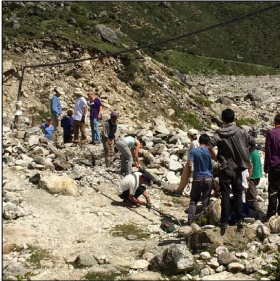
Figure 7 a) Clearing away the tower stones and releasing the main cables from the Yullajung anchorage b) Positioning large stones with the assistance of the Nepal Army.
