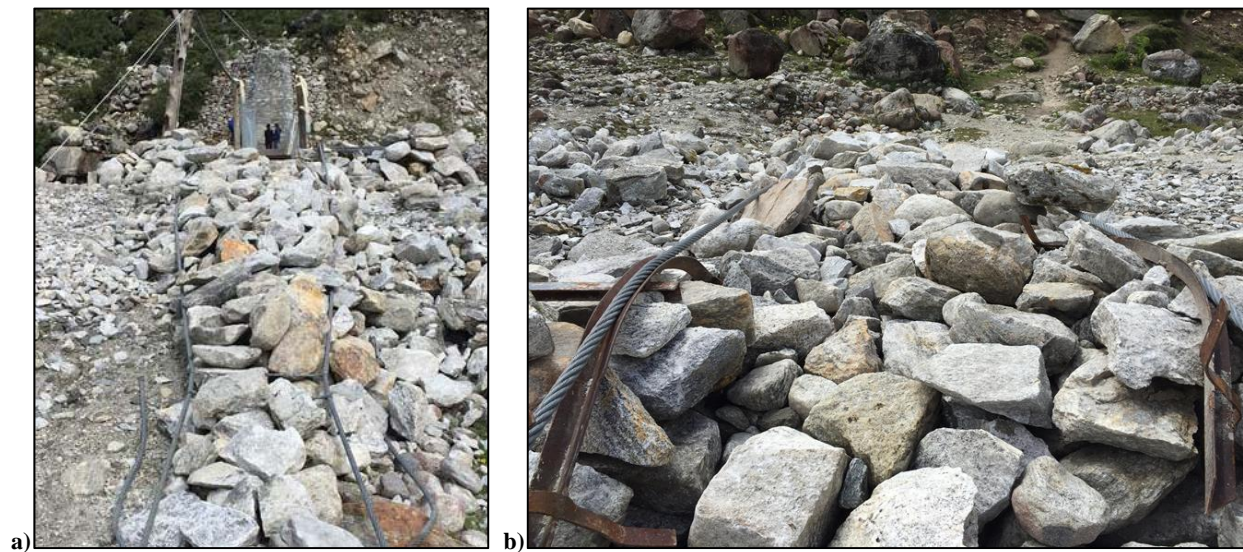
Figure 18 a) View of main cables between Yullajung anchorage and old tower location. Note the pinching of the main cables. b) Main cables at the old tower location. Note the reuse of the steel cable saddle from the old tower to ensure a large radius bend in the cables.
