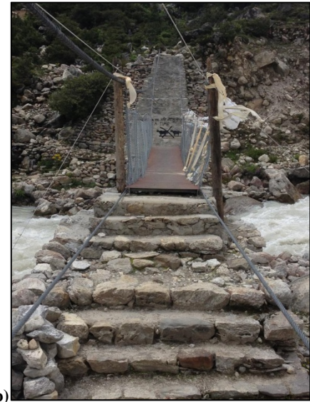
Figure 12 a) View of strengthened bridge and Thameteng abutment. b) Strengthened bridge at Yullajung abutment.
