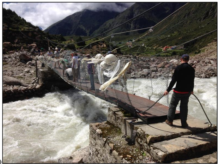
Figure 8 a) Threading the main cables through the hanger padeye loops at the deck b) Pulling the main cables through the hanger padeye loops.
