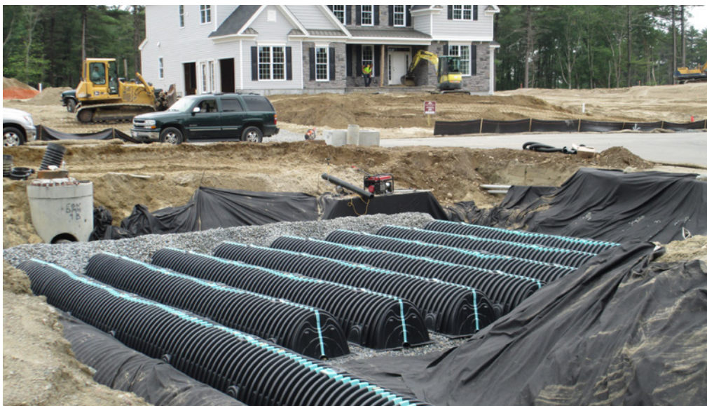
One of five CULTEC infiltration systems installed at The Preserve at Canton subdivision.
