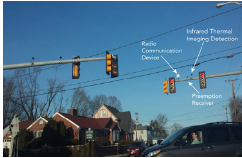
Web-based ASC system installed at each intersection sends traffic data to a remote "brain" where information is processed for sequencing.
