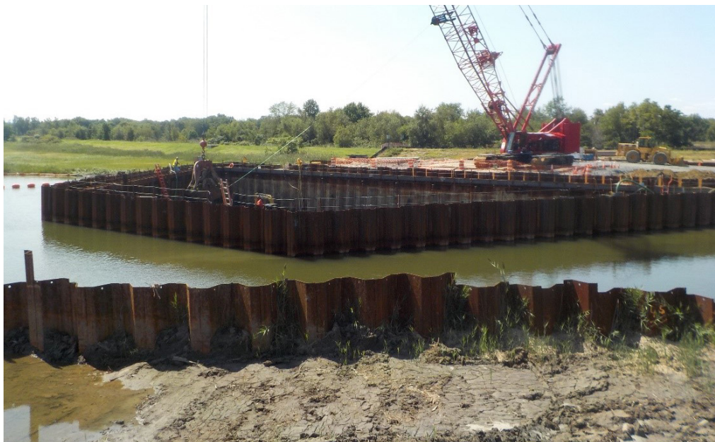
Cofferdam and diversion channel installed with excavation work ongoing.
