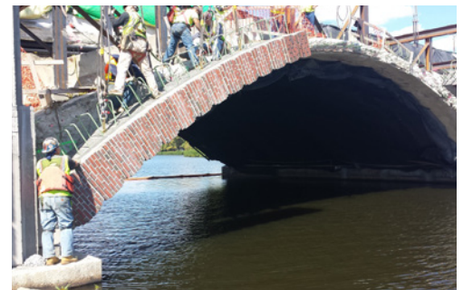
Construction of precast arch segment with brickwork
