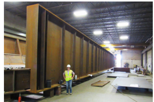
Wamsutta Bridge Girder in Fabrication: Span 3 over Acushnet Avenue was the longest at 145 feet. Each of the 3 spans required 12.5-foot deep girders to support Cooper E80 loading.
