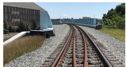
Wamsutta Railroad Track: Span 1 deck width is 35 feet wide to accommodate the curved track alignment.
