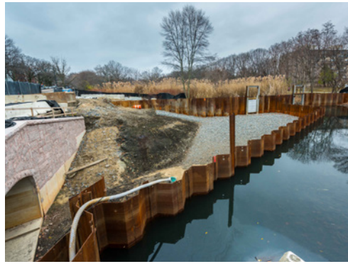
Flow restriction control structure and temporary channel separation cofferdam as seen from new Riverway culvert. Flow diverted through existing twin culverts.
