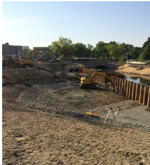
Sheet piles in place and flow diverted to right side of channel while left side is constructed.
