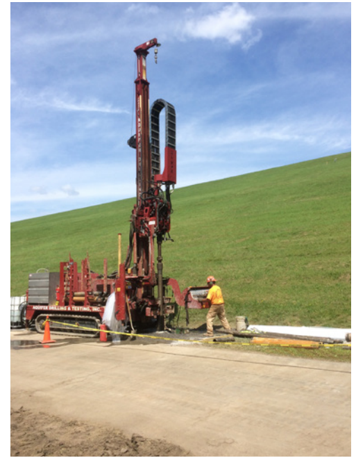
Sonic drilling for relief well installation (photo by GZA)
