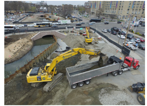
Flow diverted to right side of Muddy River while excavation proceeds on left side.
