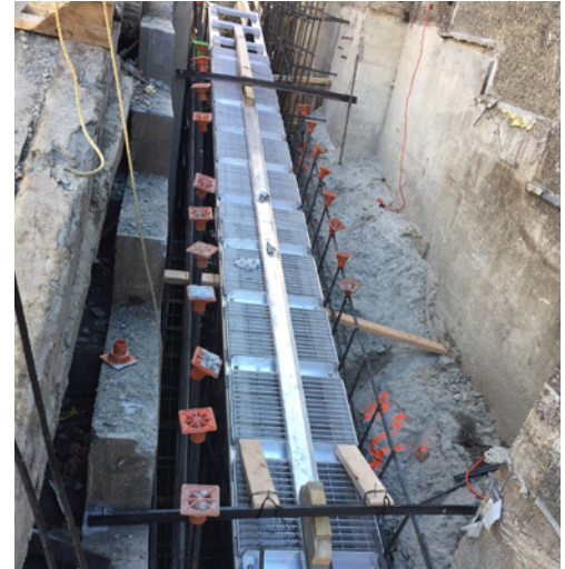
The fish ladder being installed. (Courtesy of Todd Majer)
