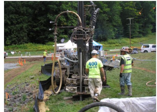
Compaction Grouting operations (photo by GZA).
