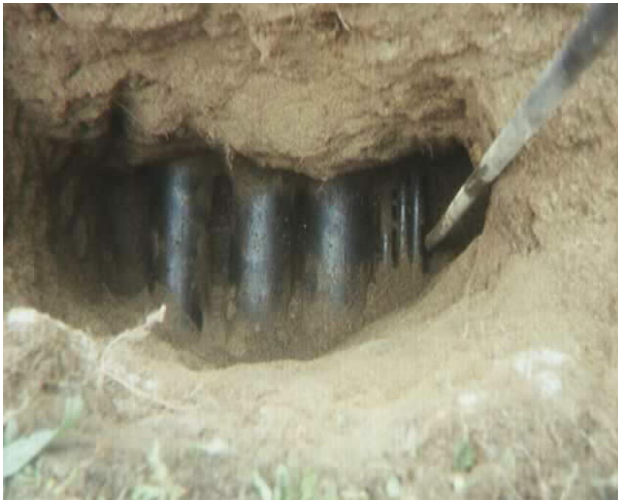
ASCE 38-02 Quality Level A. Survey grade accuracy.
