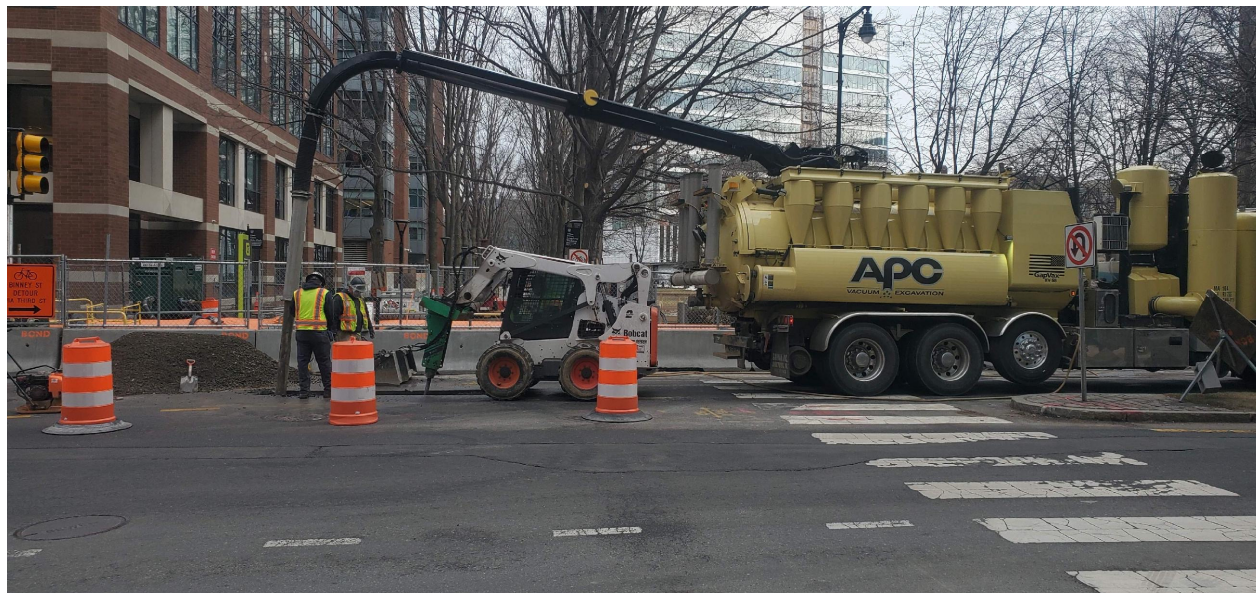
ASCE 38-02 Quality Level A. Survey grade accuracy.
