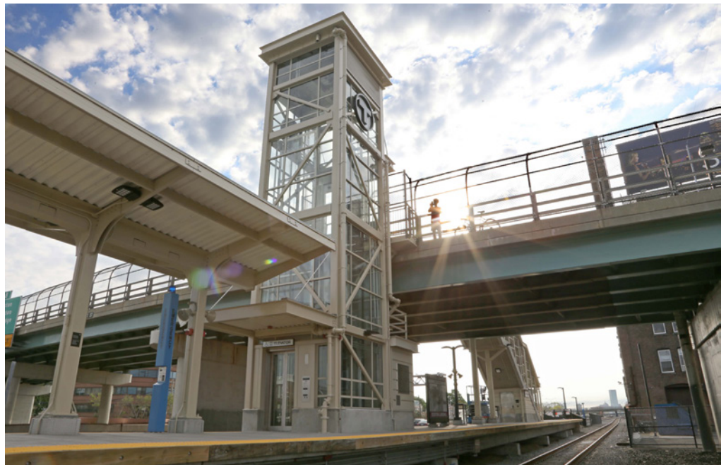
The new elevator structure at Everett Street connects the station platform to existing transportation routes.
