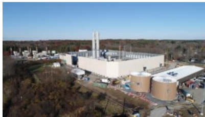
Exelon Generation Medway Peaker Project Medway, MA 200 MWs Expected online, June 2019
