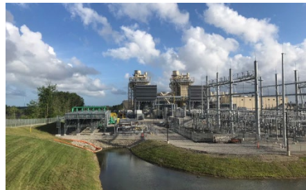
CPV Towantic Energy Center Oxford, CT 805 MWs Online June 2018
