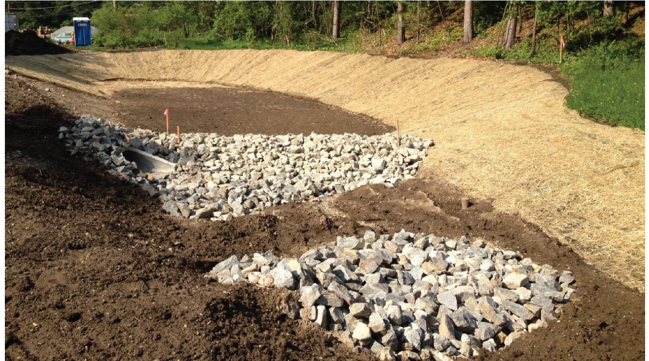
Infiltration basin under construction © MassDOT
