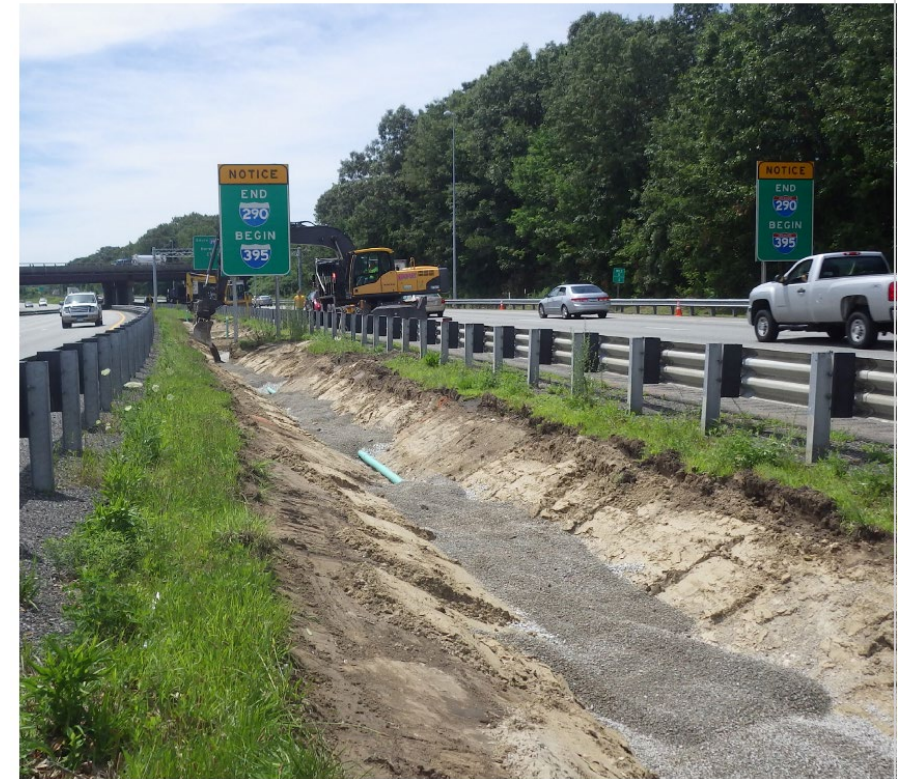
Example of a bioretention linear practice with an underdrain being installed (note the pipe within the crushed stone)
