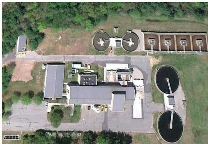
Figure 10 - The MFN Regional Wastewater Facility in Norton is managed by a regional entity that took six years to create.
