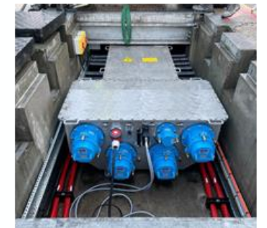
VESSEL CONNECTION 14MVA
