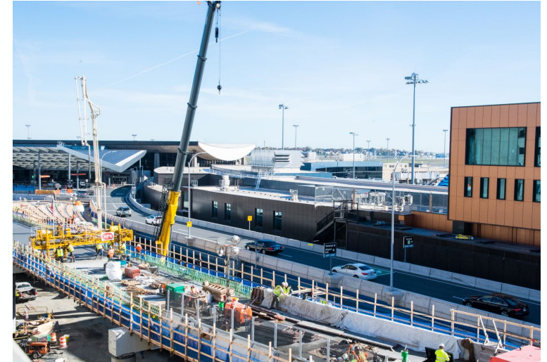
Terminal B to C Roadways
