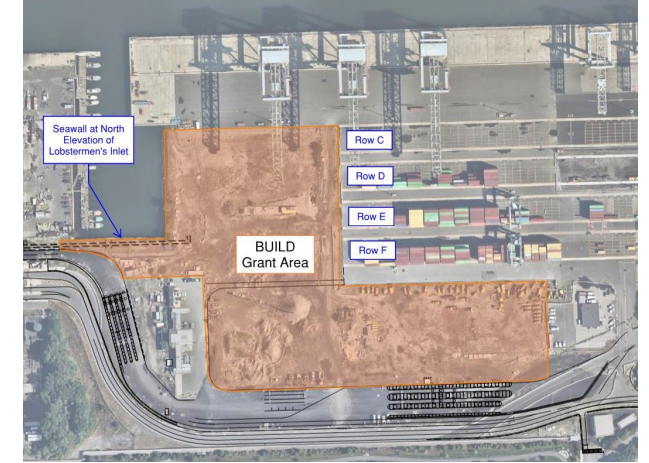
Conley Terminal Container Storage
