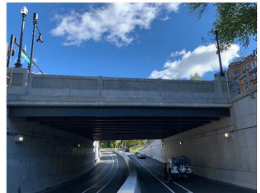
Reconstructed bridge replicated historic design features, while expanding clearance for underpass traffic.
