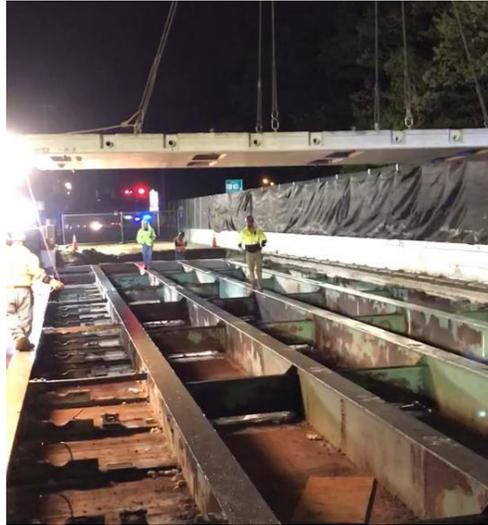
Lowering the pre-cast deck panels into place on the existing beams.
