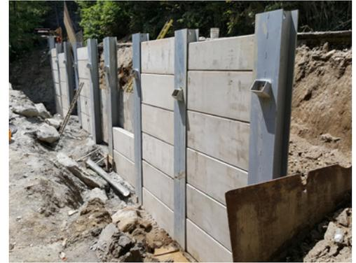
Lagging wall consisting of pre-cast concrete wall panels and soldier piles stabilize the embankment.
