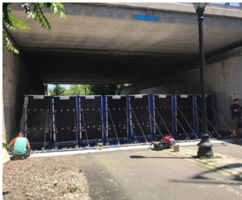
Installation of deployable flood wall on the East Boston Greenway (Image courtesy of Kleinfelder-Stoss-One Architecture)
