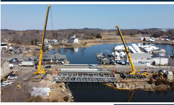
Steere performed bridge, highway, and utility design for the replacement of Bridge No. E-11-001 (2TV) carrying Main Street over the Essex River in Essex, MA. The project included a superstructure replacement and substructure rehabilitation, requiring a temporary bypass road during construction including a temporary bridge and numerous utility relocations. The replacement was performed under the MassDOT Footprint Bridge Program.
