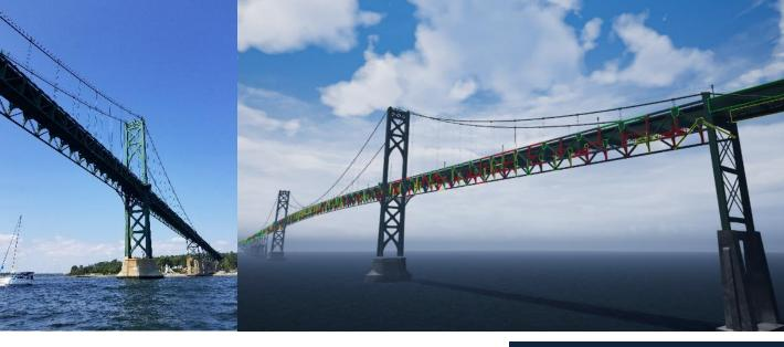
Steere Engineering Inc. utilized 3D modeling for the creation of a Virtual Reality Simulation of the Mt. Hope Bridge. The base model was developed from the original drawings of the bridge from the 1920's. The model was then optimized for Virtual Reality and connected to the current bridge inspection report. This provided a realistic environment of the bridge with all the valuable information attached to each element for a variety of uses.
