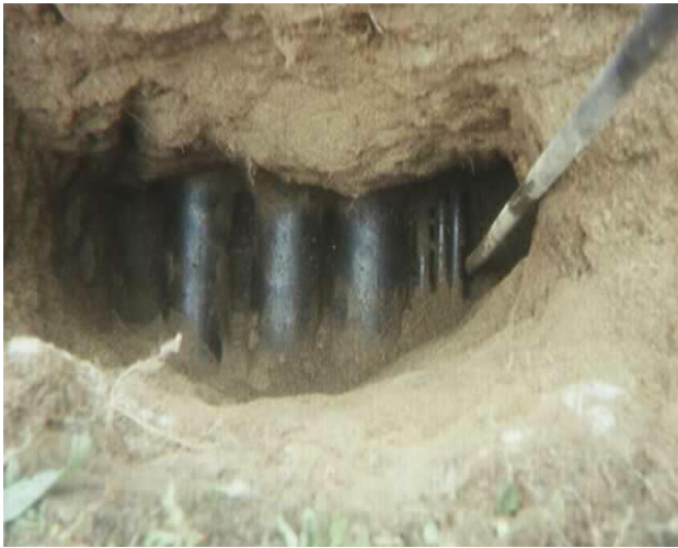
ASCE 38-02 Quality Level A. Survey grade accuracy.
